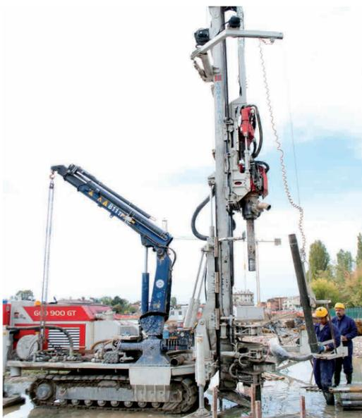
High-performance hydraulic drilling rig with double head system able to fulfil:
