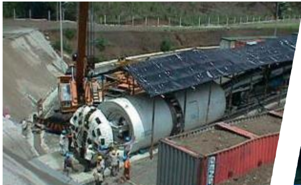
TBM HEAD + SHIELD
