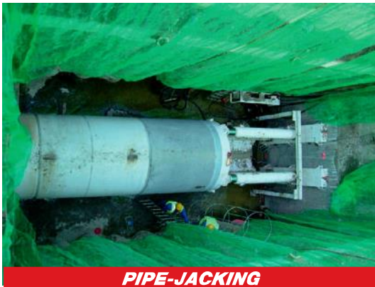
OPEN SHIELD OPERATION
