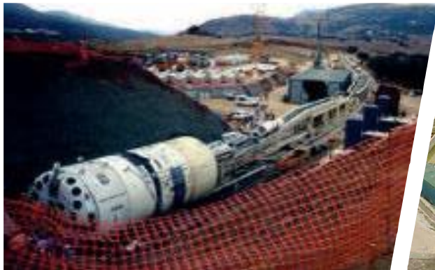
TBM BACK UP
